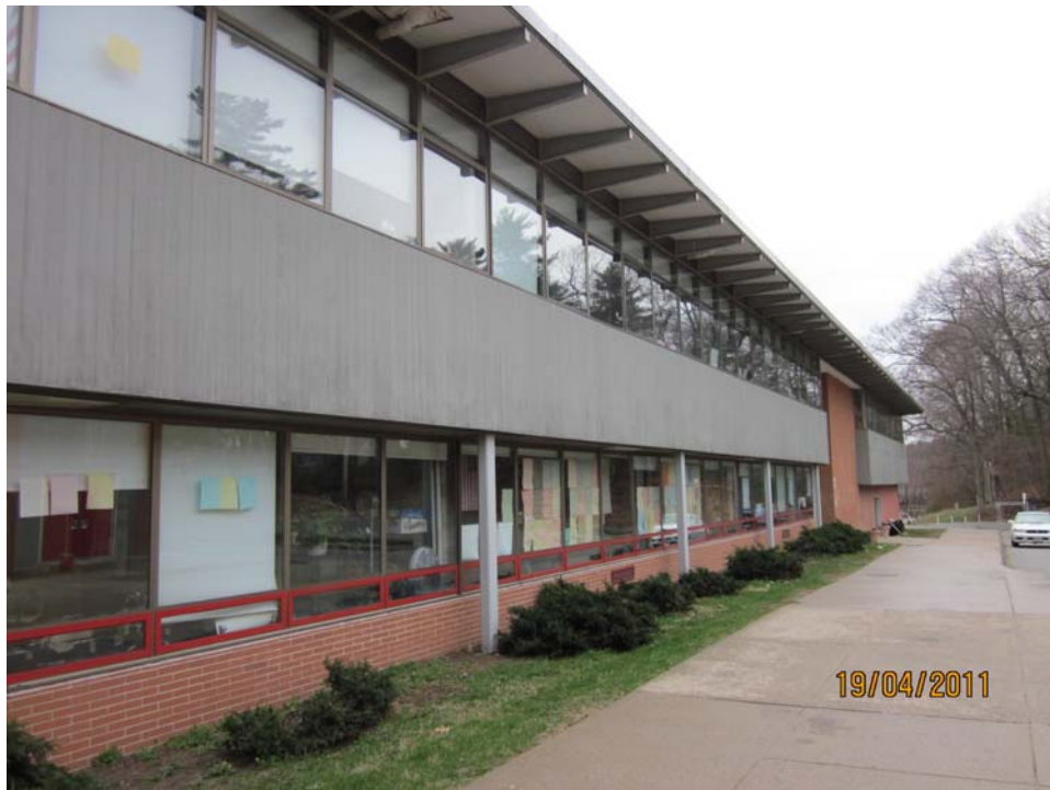
Photo 16: Condition of two story academic wing.
