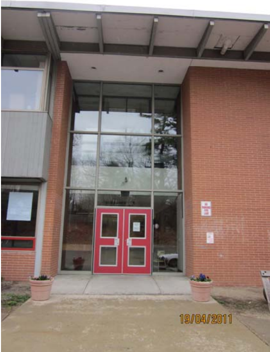
Photo 17: Two story curtain wall at door.
