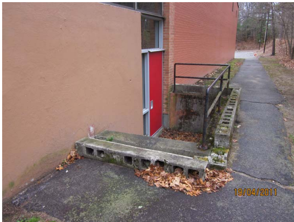
Photo 12: Areaway condition at southwest corner.
